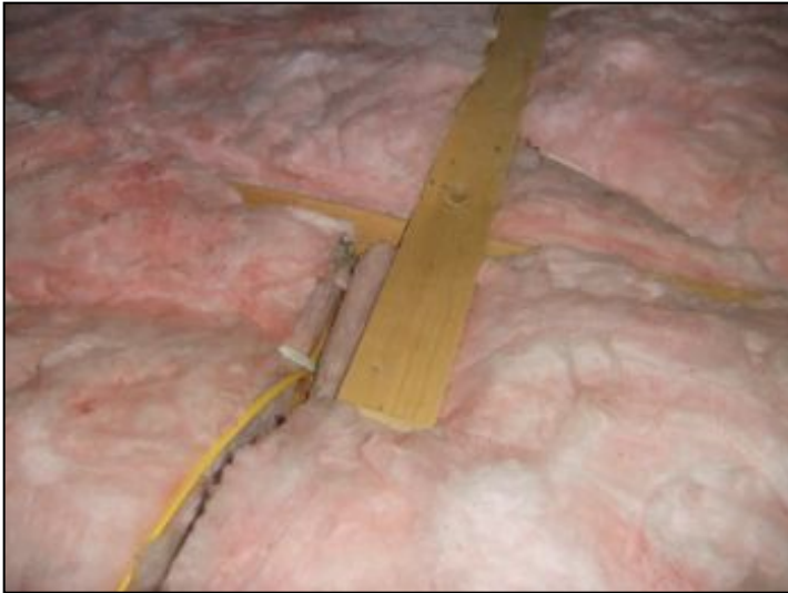
ROOF & ATTIC INSULATION CONDITION
