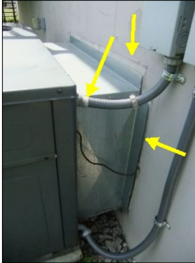
Reseal ductwork to house and reattach conduit nut
