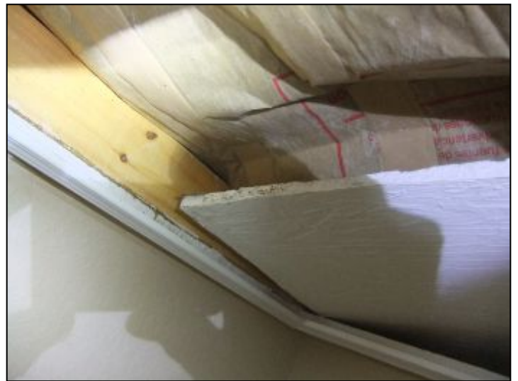
Attic access condition
