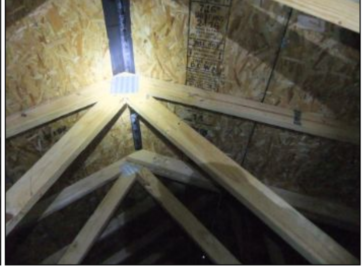
Ridge vent and sheathing clips present
