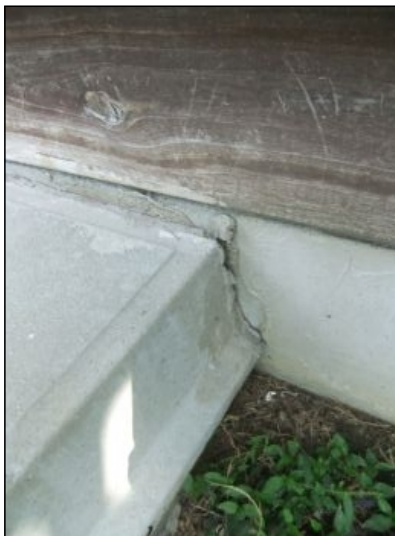
step slopes to house
