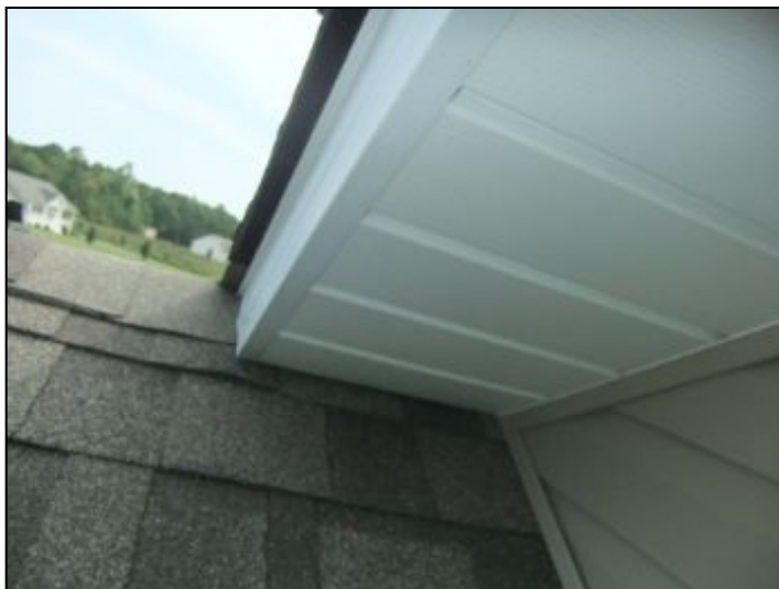
ROOF & ATTIC ROOF CONDITION
