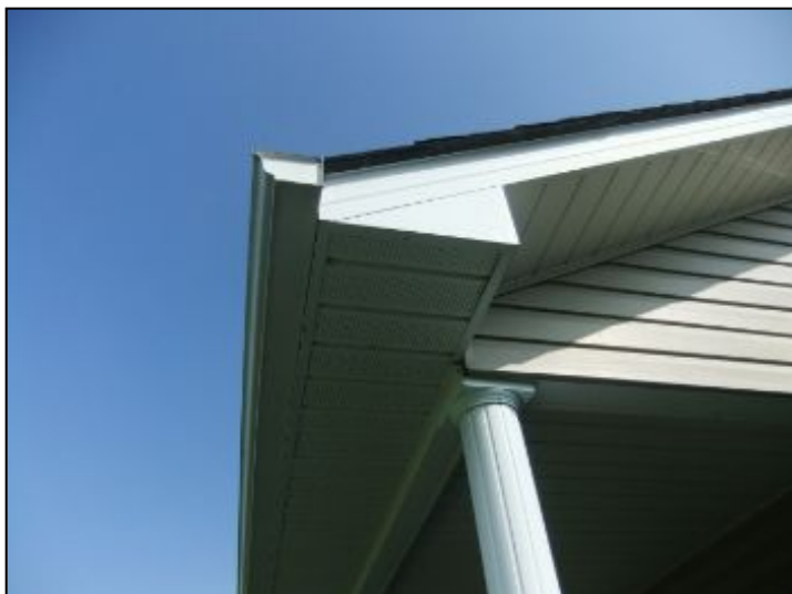
ROOF & ATTIC SOFFIT AND FASCIA
