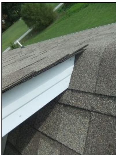
ROOF & ATTIC FLASHING
