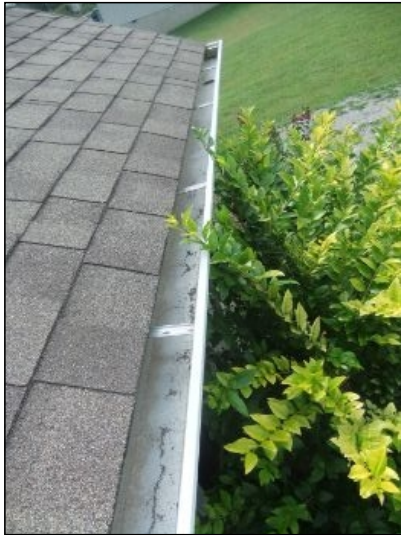
ROOF & ATTIC RAIN GUTTERS AND DOWNSPOUTS CONDITION
