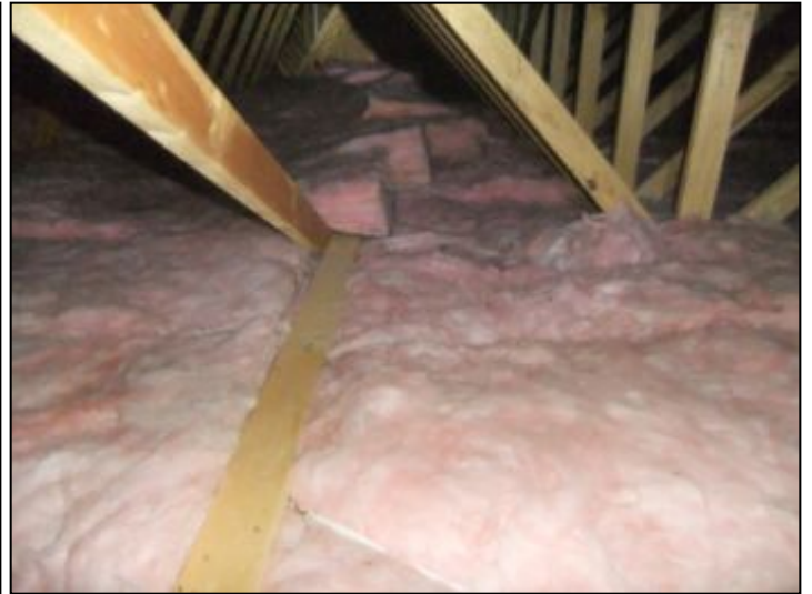
ROOF & ATTIC INSULATION CONDITION
