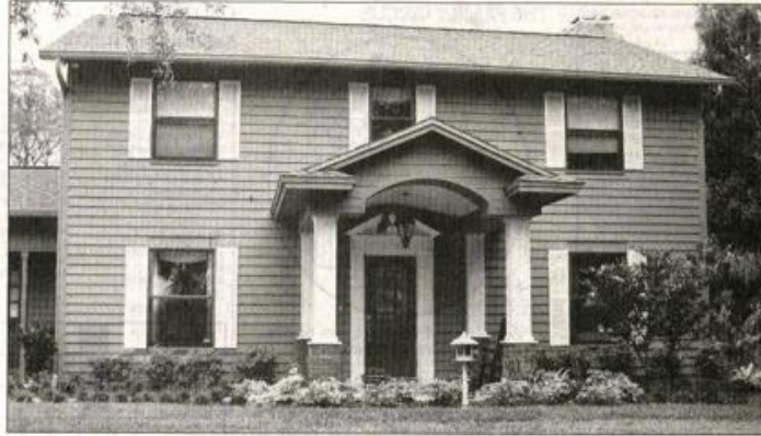
SPECIAL TO THE NEWS-PRESS ■ The Hutchcraft family of Fort Myers added this front porch to their home.
